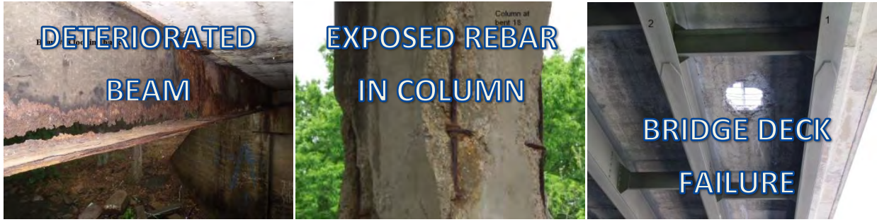
Figure 1. Deteriorating Bridges in Arkansas
