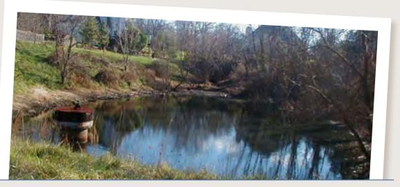
Figure 2. Typical stormwater management pond showing overflow riser.
