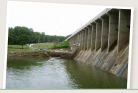
Brighton Dam: a slab and buttress dam
