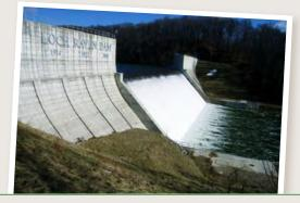
Loch Raven Dam: a concrete gravity dam
