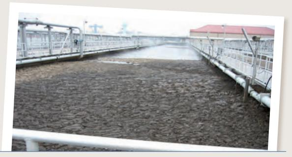
Figure 1. Sludge and scum accumulation at the Back River Wastewater Treatment Plant.
