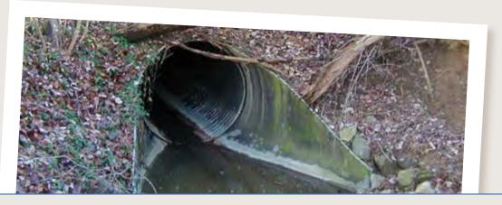
Figure 1. Typical stormwater outfall to natural stream.
