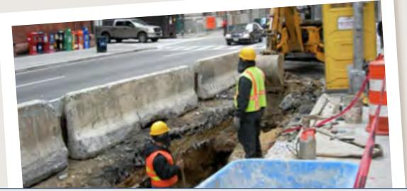
Figure 1. Crews repairing leaking water mains in Baltimore City (Source: KCI, 2010)
