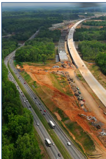
Figure 3. I-85 Yadkin River Bridge, Photo Courtesy of NCDOT
