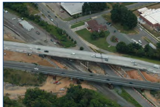
Figure 10. US 52 Bridge Replacement, Photo Courtesy of NCDOT
