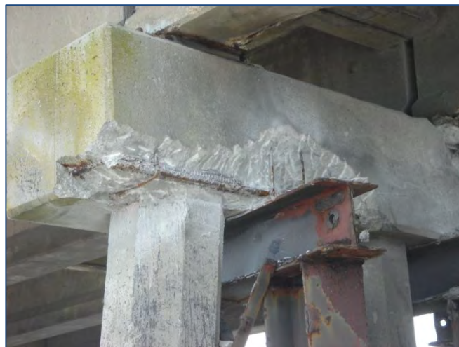
Figure 5. Bonner Bridge Repairs, Photo Courtesy of NCDOT
