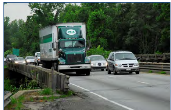
Figure 7. I-85 Bridge over Railroad, Photo Courtesy of NCDOT
