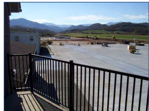
Figure 2. Macon County Airport Ramp Reconstruction
