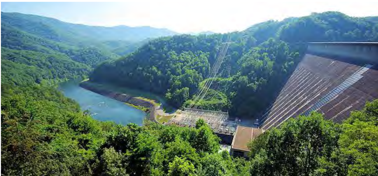
North Carolina Section Historic Civil Engineering Landmark - Tennessee Valley Authority Fontana Dam, Fontana, NC
