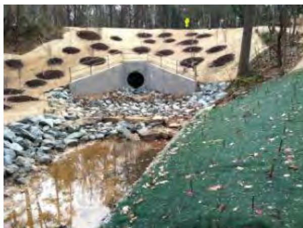
North Hills Drive Culvert Repair, City of Raleigh, 2012
