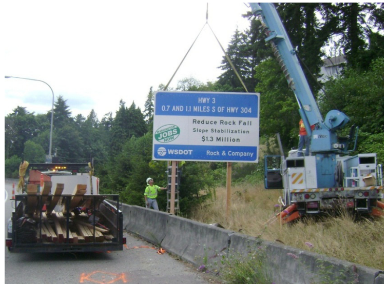
Road maintenance; Courtesy: WSDOT
