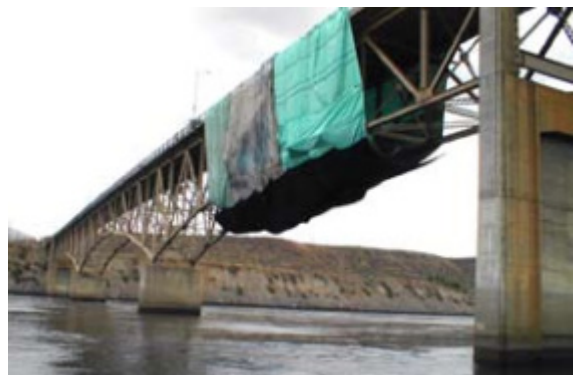
Columbia River Bridge in Bridgeport undergoing steel repainting; Courtesy: WSDOT.
