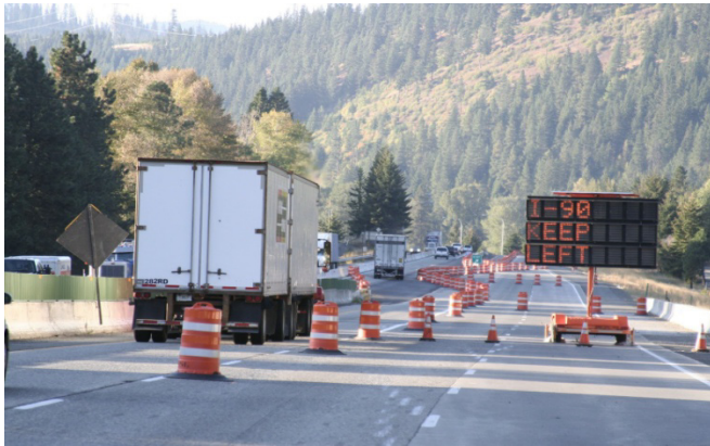
I-90 Construction; Courtesy: WSDOT
