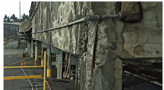
Magnolia Bridge, Seattle, Washington, has a SR of only 18; Courtesy: KIRO 7
