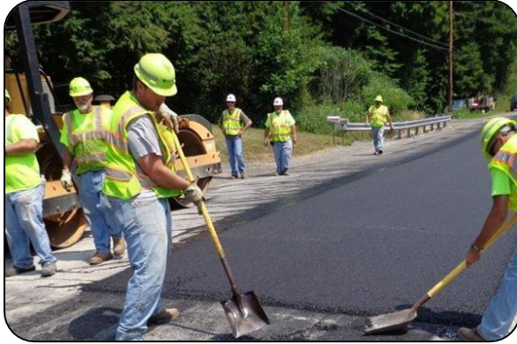
Road and Bridge Construction Workers Picture from PennDOT Local Technical Assistance Program
