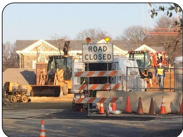
Bridge Closed for Repair and Maintenance Picture Courtesy of Intelligent Infrastructure Systems (IIS)
