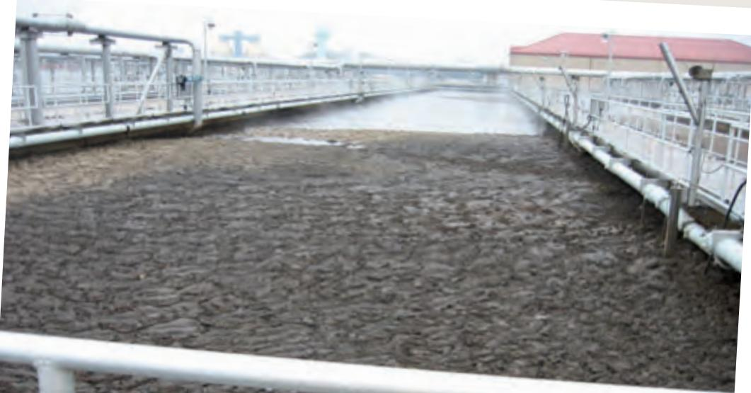
Figure 1. Sludge and scum accumulation at the Back River Wastewater Treatment Plant.
