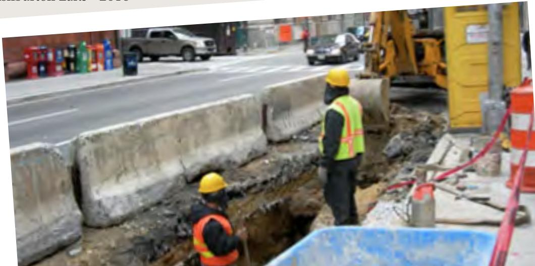
Figure 1. Crews repairing leaking water mains in Baltimore City (Source: KCI, 2010)
