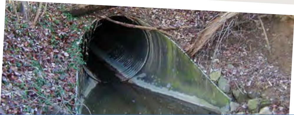
Figure 1. Typical stormwater outfall to natural stream.
