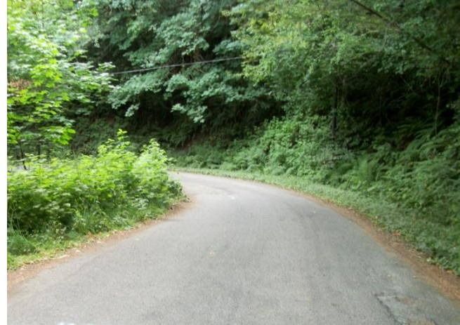
Figure 10. Butler Valley Road has a PCI of 60, representative of the overall grade in Humboldt County
