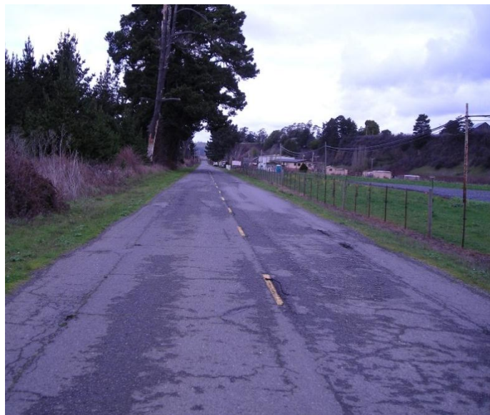
Figure 2. Existing asphalt concrete deteriorating on Eel River Drive near Fortuna, CA.
