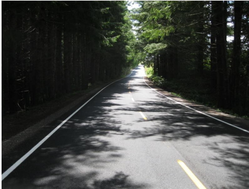
Figure 11. A section of Bald Hills Road following paving in 2012; This road provides an alternative access between the Wietchpec and Orick (HWY 101).
