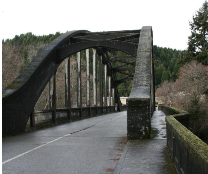
Figure 1. Bridge over North Fork Mad River near Korbel, CA
