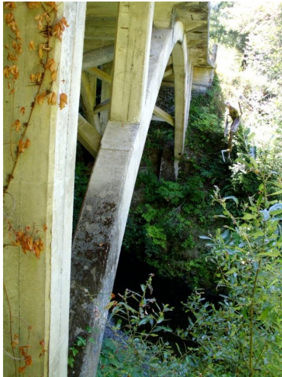
Figure 12. Concrete Spandrel Arch Bridge Over the Mattole River
