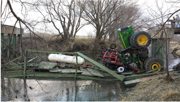
Photo 2- Rural bridge failure
