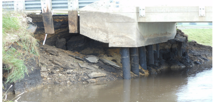
Photo 3- Bridge abutment damage due to scour
