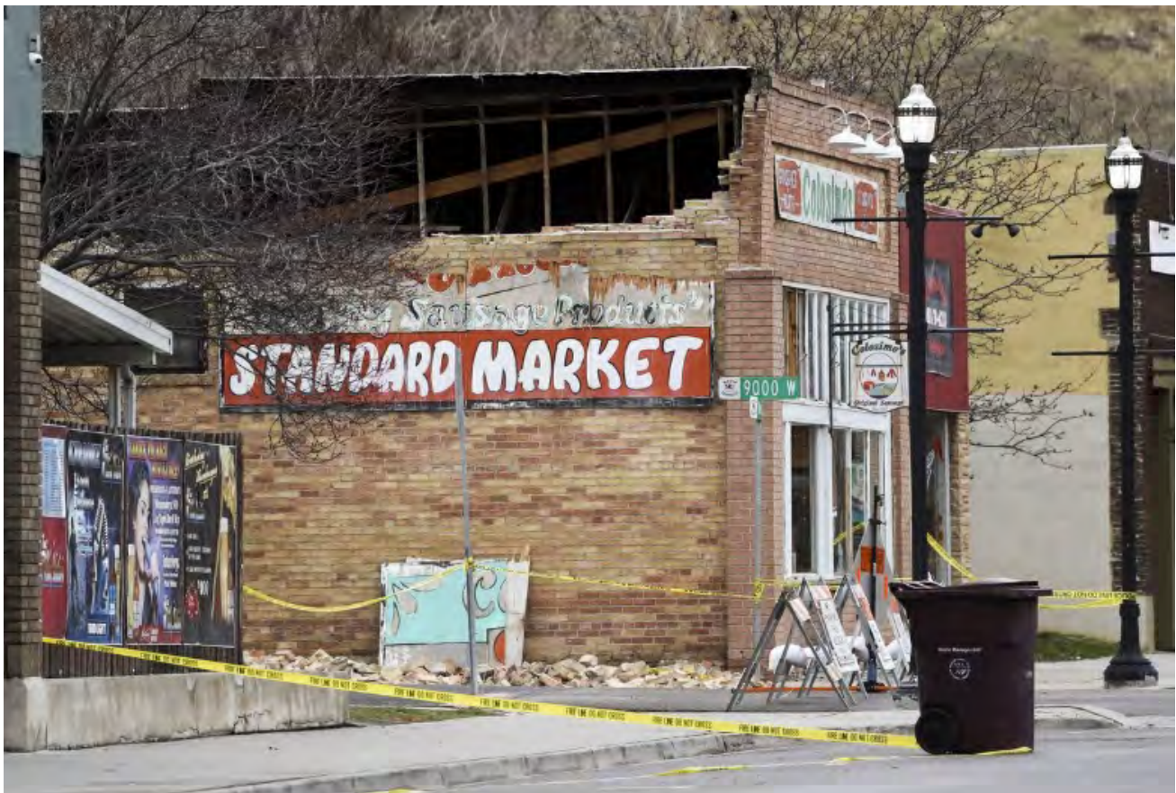
Figure 1 – Photo of damaged masonry structure that shutdown local business (Deseret News, 2020b.)
