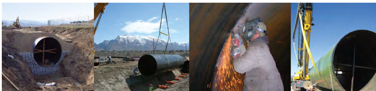
Figure 3 – PRCEP construction (PRWUA, 2020)
