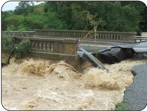
Damage to a Bridge due to Flood Picture Courtesy of PennDOT
