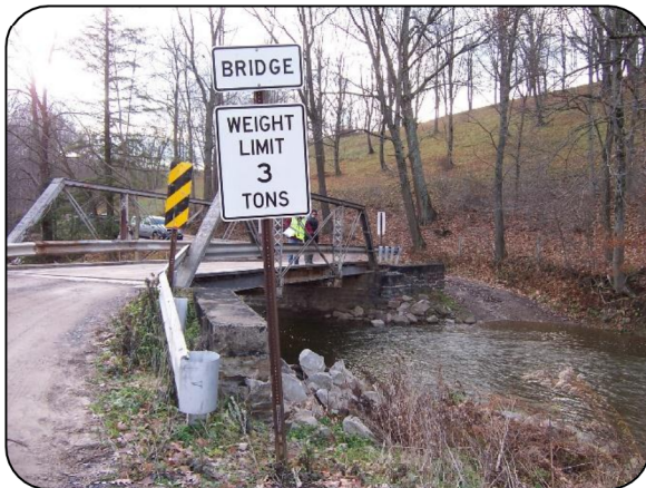
Weight Restriction on a Structurally Deficient Bridge Picture Courtesy of Gannett Fleming, Inc.
