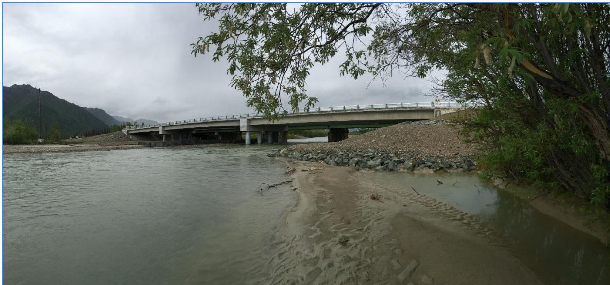
Structurally deficient bridges are being replaced, like at the Tok River on the Tok Cutoff. The old bridge in the background was demolished after the new one was opened. These timely replacements are key to keeping bridge infrastructure from falling into disrepair.
