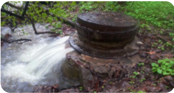
Figure 3 – Wet weather sanitary sewer overflow (Source: Blue Water Baltimore)
