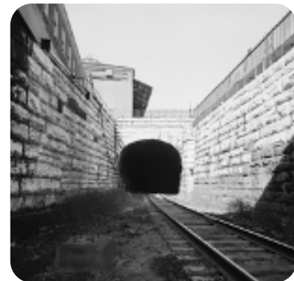
Figure 2 – South approach to Howard Street Tunnel (courtesy of National Park Service)
