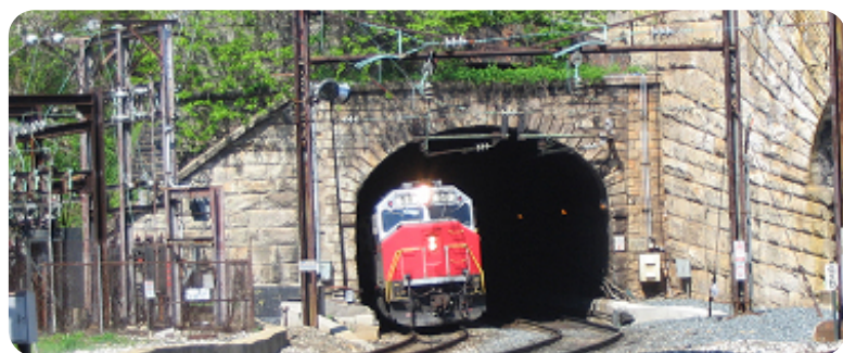
Figure 4 – B&P Tunnel (courtesy of MDT)
