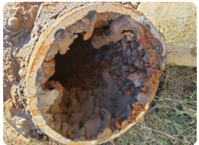
Figure 1 – City of Bowie cast iron water main
