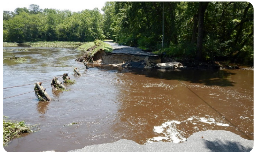
Figure 2 – Barren Creek Pond dam failure (July 14, 2016)
