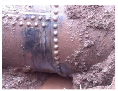
The condition of the drinking water infrastructure in the City of Duluth is poor. The City has 433 miles of piping. Durable cast-iron pipe, as shown in the above photo, was installed in the 1880s and 1890s and can last for 120 to 130 years, meaning it is now coming to the end of its design service life. The piping installed from 1910 to 1920, projected to last about 100 years, is also due to be replaced. Pipe installed in the 1960s and 1970s, which has had a life span of 50 to 60
