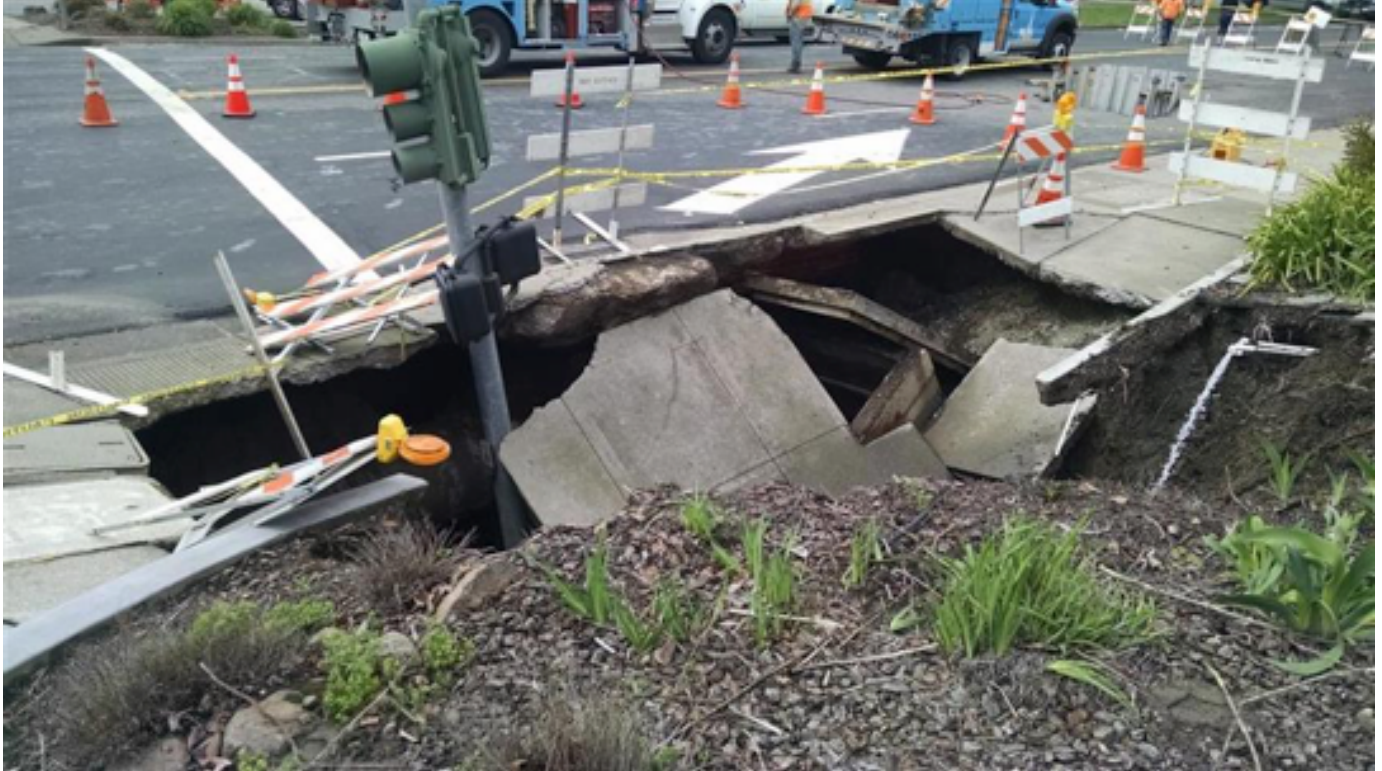
TOWN OF MORAGA, CALIFORNIA SINKHOLE THAT FORMED IN MARCH OF 2016 DUE TO THE FAILURE OF AN UNDERGROUND 96-INCH DIAMETER STORM DRAIN PIPE. THE SINKHOLE GREW TO A DEPTH OF 15 FEET AND WAS AFFECTIONATELY REFERRED TO AS “SINKY THE SINKHOLE” BY THE LOCAL RESIDENCE OF THE TOWN.
